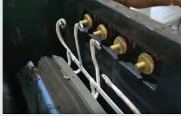
Fig. n: Assembly in the transformer tank
