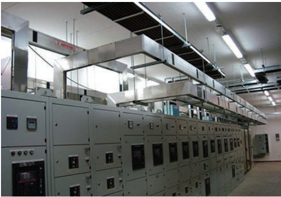
Fig. 2.11: Industrial application of a busway
