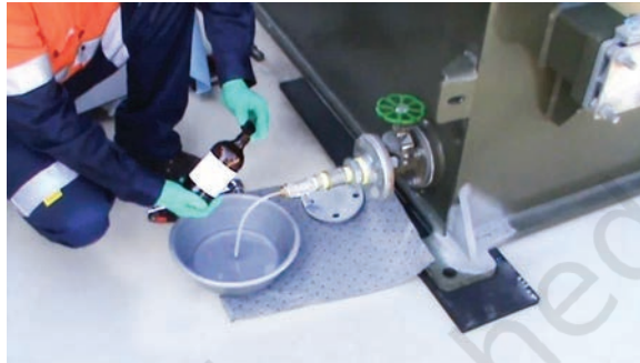
Fig. 11.22: Draining oil from a transformer
