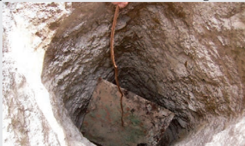
Fig. c: Placing a copper plate in the pit
