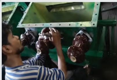
Fig. l: Fitting high voltage bushing on the transformer
